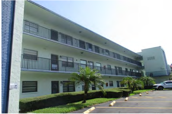
41 Exterior Building Overview
