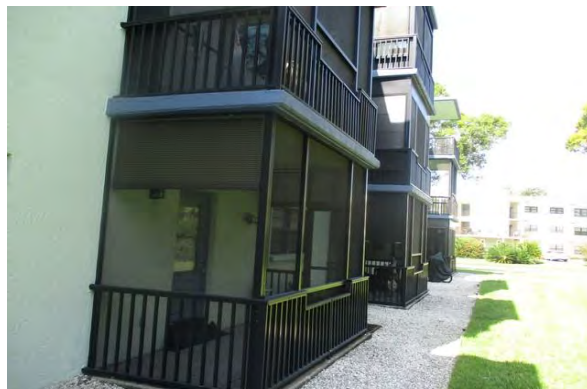
39 Exterior Balcony Overview
