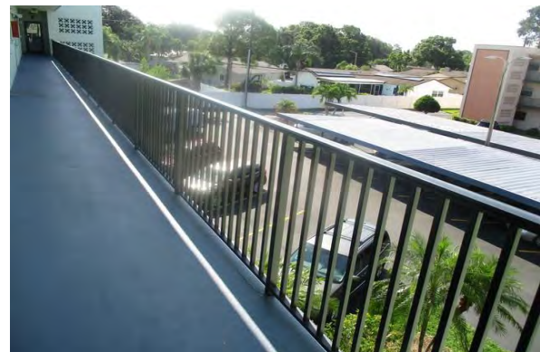
32 Walkway Railings Overview
