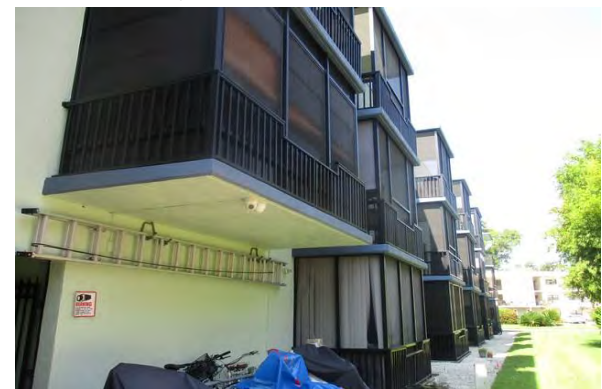
38 Exterior Balcony Overview
