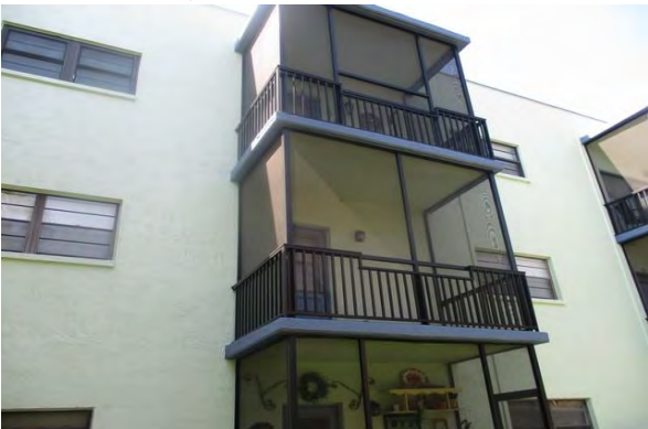
37 Exterior Balcony Overview
