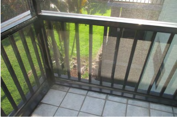
19 Interior Balcony Overview
